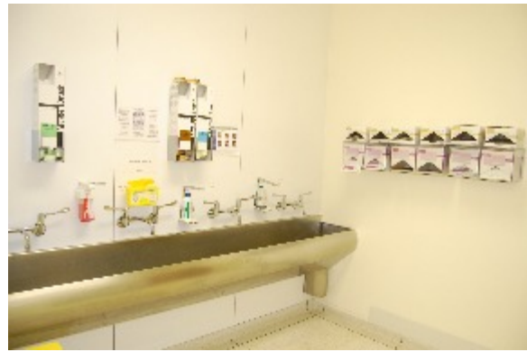
The scrub room. It is equipped with elbow operated taps. There are dispensers on the wall containing disposable nail brushes and sponges impregnated with chlorhexidine, PCMX or iodine and separate dispensers. Sterile gloves are on the wall.
