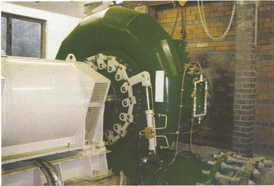
Figure 5.17 The 450 kW horizontal-axis Francis turbine of a small-scale plant in Scotland, commissioned in 1993. The inflow (at lower right) is 2.1 \text{ m}^3 \text{ s}^{-1} at a head of 25 m. The turbine, rotating at 750 rpm, drives the generator whose casing can be seen on the left
