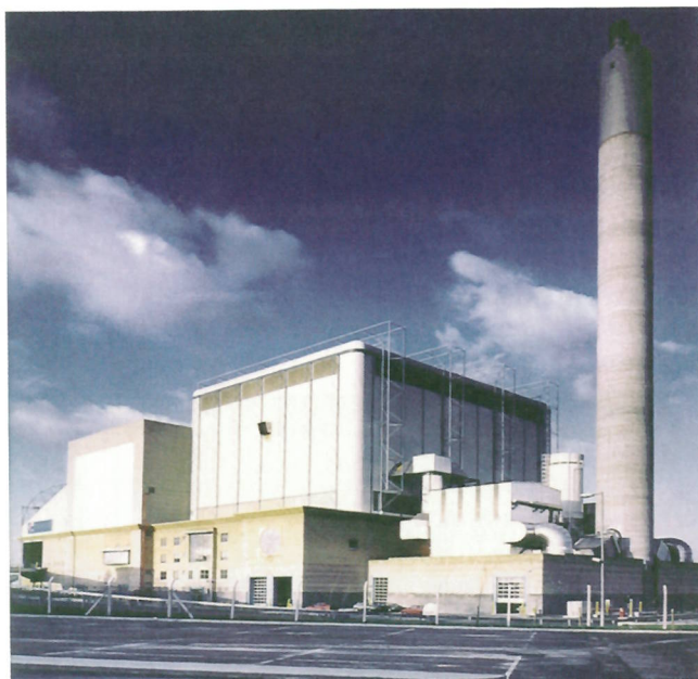
Figure 4.11 The SELCHP (South-East London Combined Heat and Power) plant, commissioned in 1984, is designed to incinerate 420 000 tonnes of MSW per year, producing steam for a 31 MW turbo-generator and heat for a local district heating scheme
