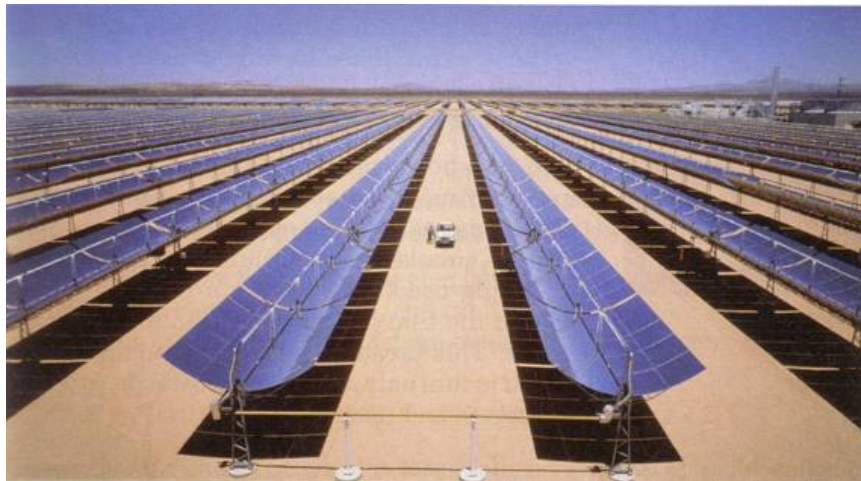
SEGS solar collector field at Kramer Junction, California (source: Boyle, G., Renewable Energy (2000))
