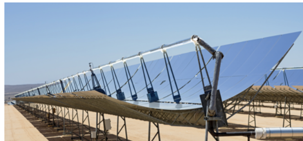
Figure 5 - Parabolic trough in series [12]
