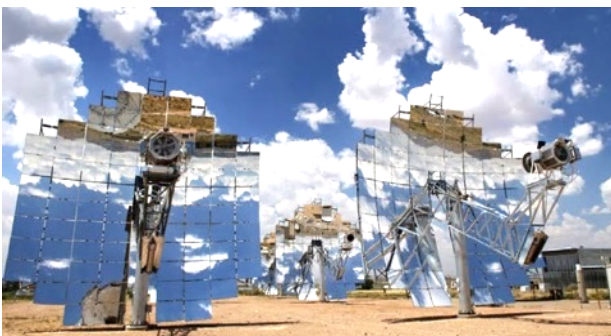
Figure 10 - Multiple solar dishes coupled with their respective heat engines [8].
