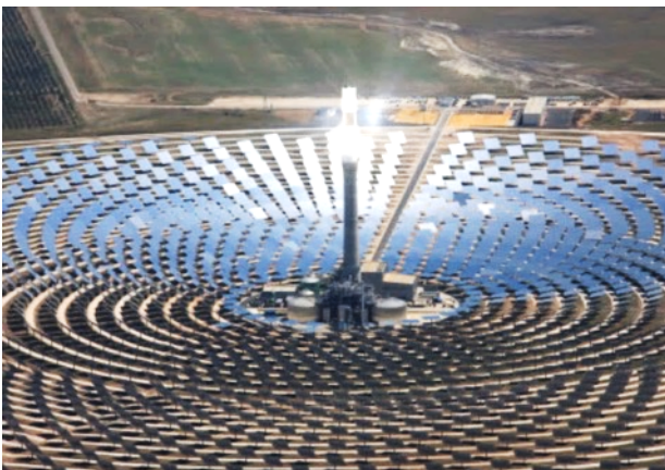
Figure 7 - Solar tower field with central receiver [13]
