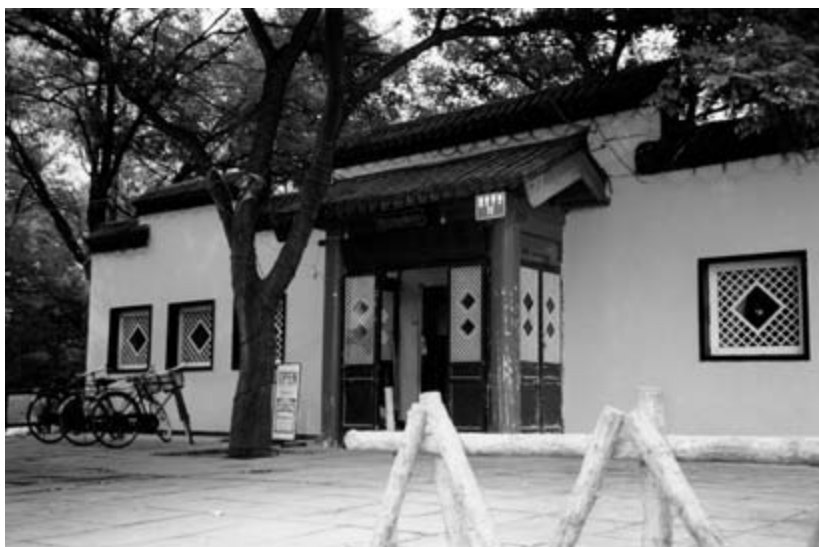
The Yellow Pavilion, the base for a cineclub near the Beijing Film Academy. (Photo by Zhang Zhen)
